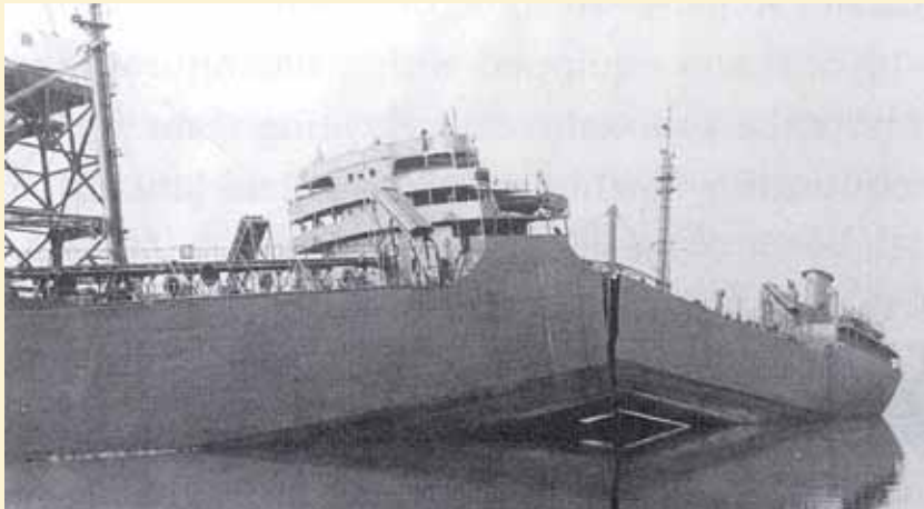
A number of WW2 Liberty ships failed due to cracks being able to run through a welded structure, where before they would have been stopped in a riveted ship. So the stress concentration at a hatch corner caused complete failure.
